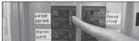
Figure 27 - Circuit Breaker
