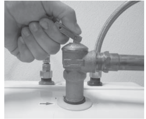
Figure 31 - T&P Relief Valve
