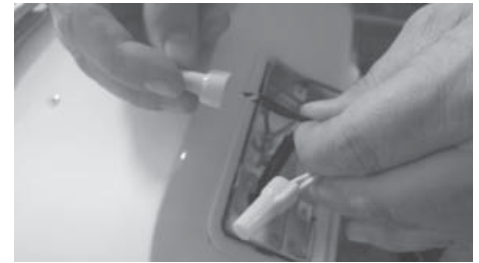
Figure 18 - Connecting the electrical wires.
